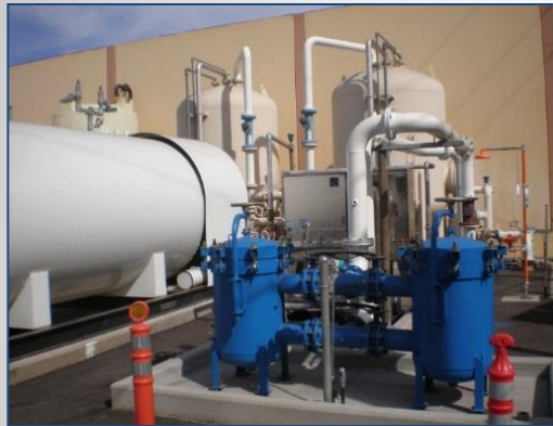
Weak-Base Anion Exchange (WBA)
