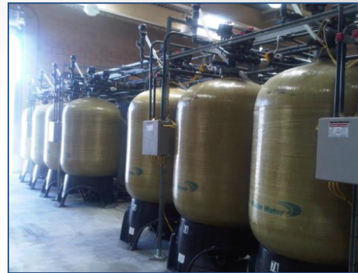
Strong-Base Anion Exchange with Residuals Treatment (SBA)
